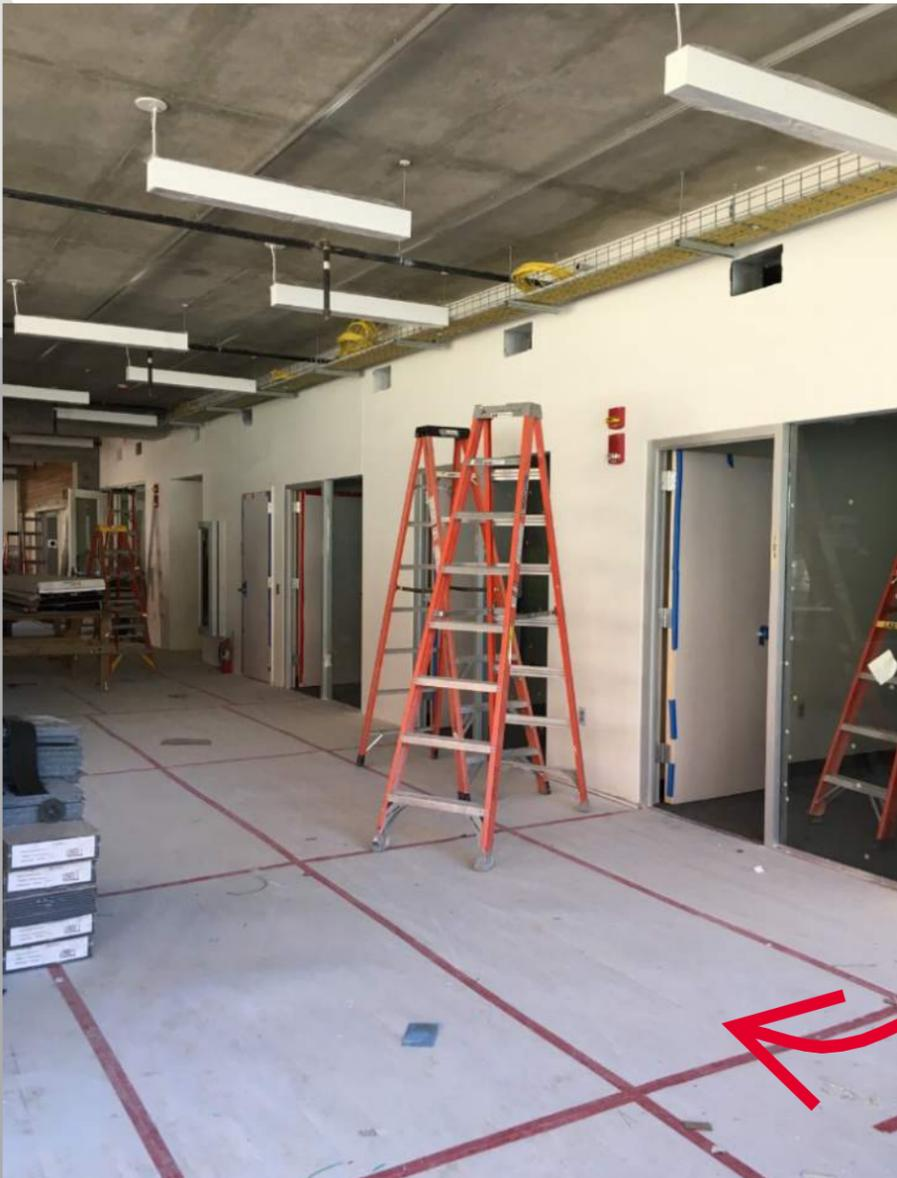
**EXPOSED CONCRETE FLOORS STILL NEED TO BE POLISHED (CURRENTLY COVERED BY FLOOR PROTECTION)**
