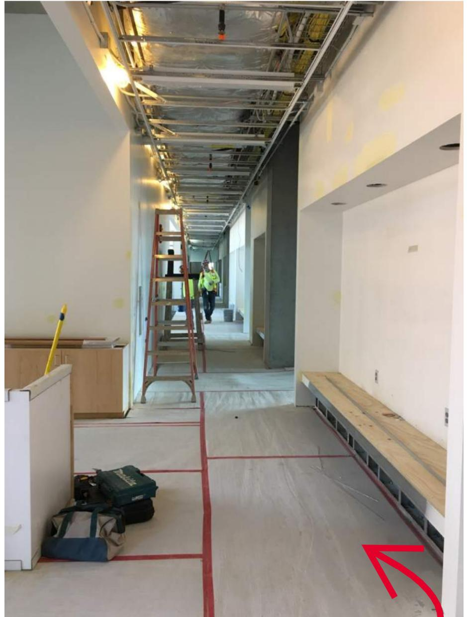
**BARTLETT ACADEMIC SUCCESS CENTER LEVEL 3 LOBBY AND HALLWAY ARE NEARLY COMPLETE AND READY FOR FLOOR PROTECTION TO BE REMOVED AND CONCRETE TO BE POLISHED! WOOD SLATTING IS BEING FITTED AT ELEVATOR FRONTS - BEFORE BEING REMOVED AND ETCHED WITH THE FLOOR DESIGNATION!**
