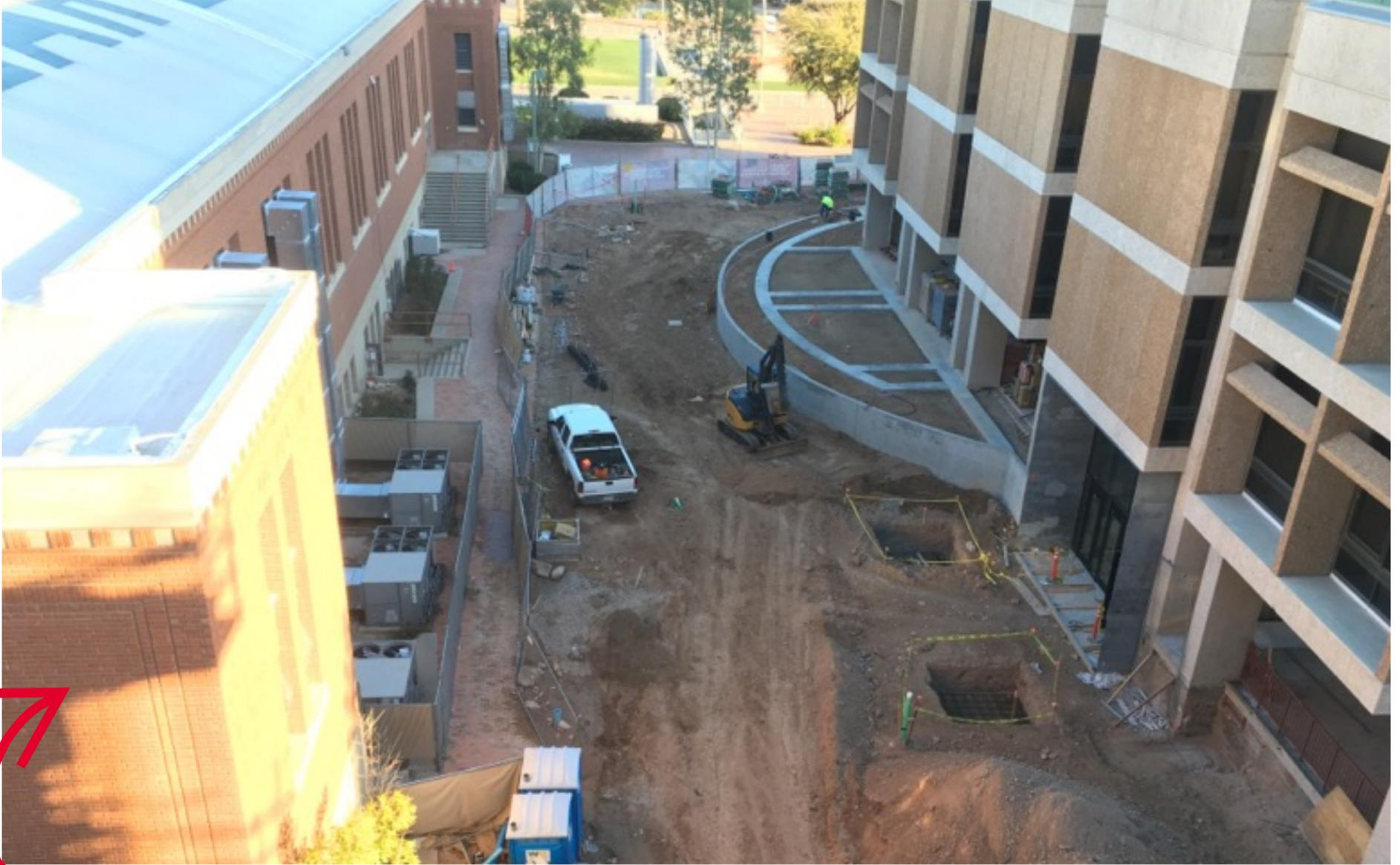
THE MAIN LIBRARY WEST PATIO WORK IS PROGRESSING WITH INSTALLATION OF CONCRETE BANDS. THE BRICKS WILL COME NEXT! VIEW IS FROM THE ROOF OF THE NEW STUDENT SUCCESS BUILDING.
