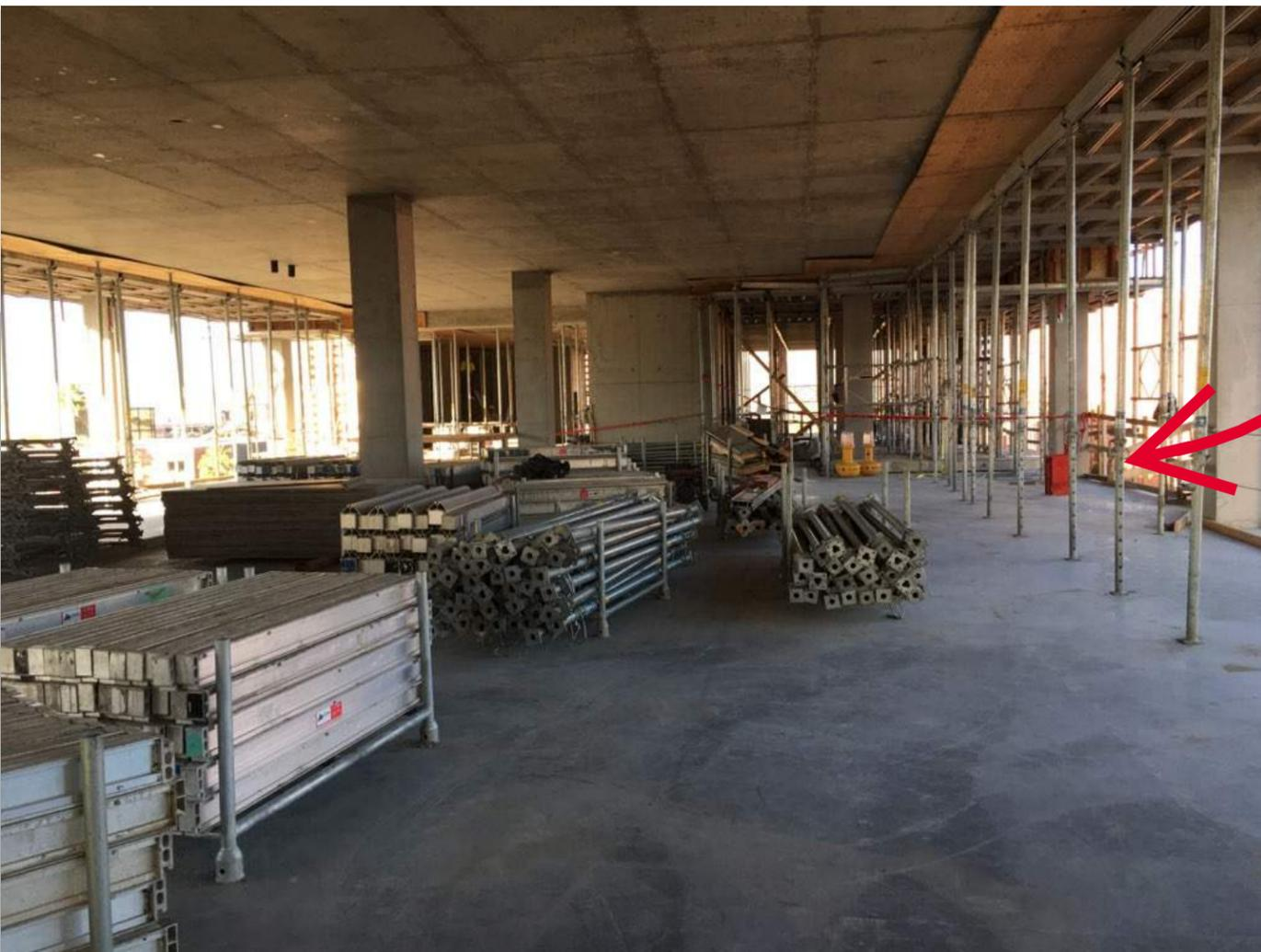
STUDENT SUCCESS BUILDING LEVEL 4 FORMWORK IS BEING STRIPPED!
