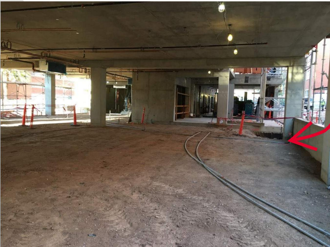
STUDENT SUCCESS BUILDING LEVEL 1 IS BEING PREPARED FOR SLAB ON GRADE PLACEMENT WITH UNDERGROUND UTILITIES AND GRADING
