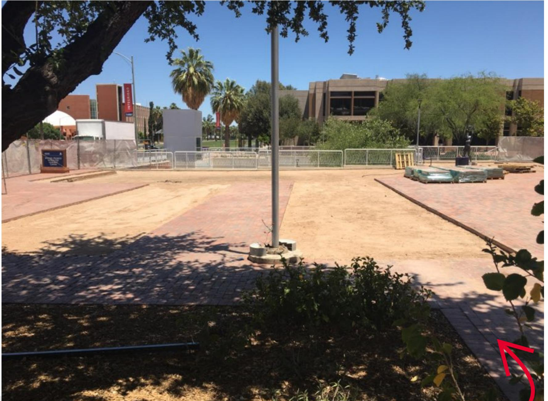
VIEW OF HARDSCAPE WORK TO THE NORTH OF MAIN LIBRARY POD 'A'. BRICK HAS BEEN REMOVED FOR NEW CONCRETE BANDS TO BE INSTALLED
