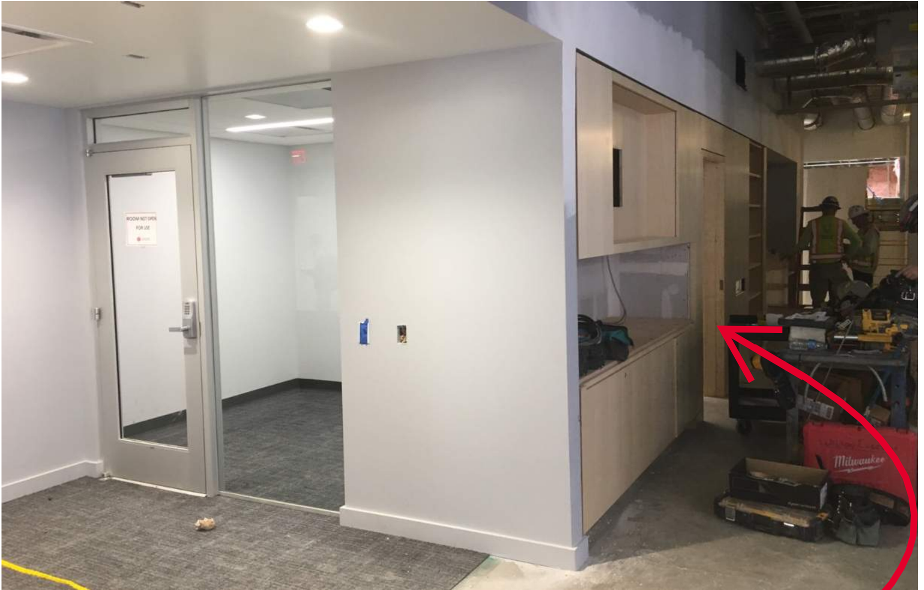
SCIENCE & ENGINEERING LIBRARY SERVICE POINT MILLWORK IS BEING INSTALLED!
