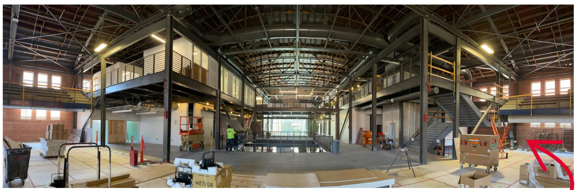
*Inside the main entrance standing on the historic gym floor, looking south. Interior windows are going in on level 3, electrical light fixtures are hanging from the level 2 ceiling, and the bathroom partitions are going in on level 1.*
