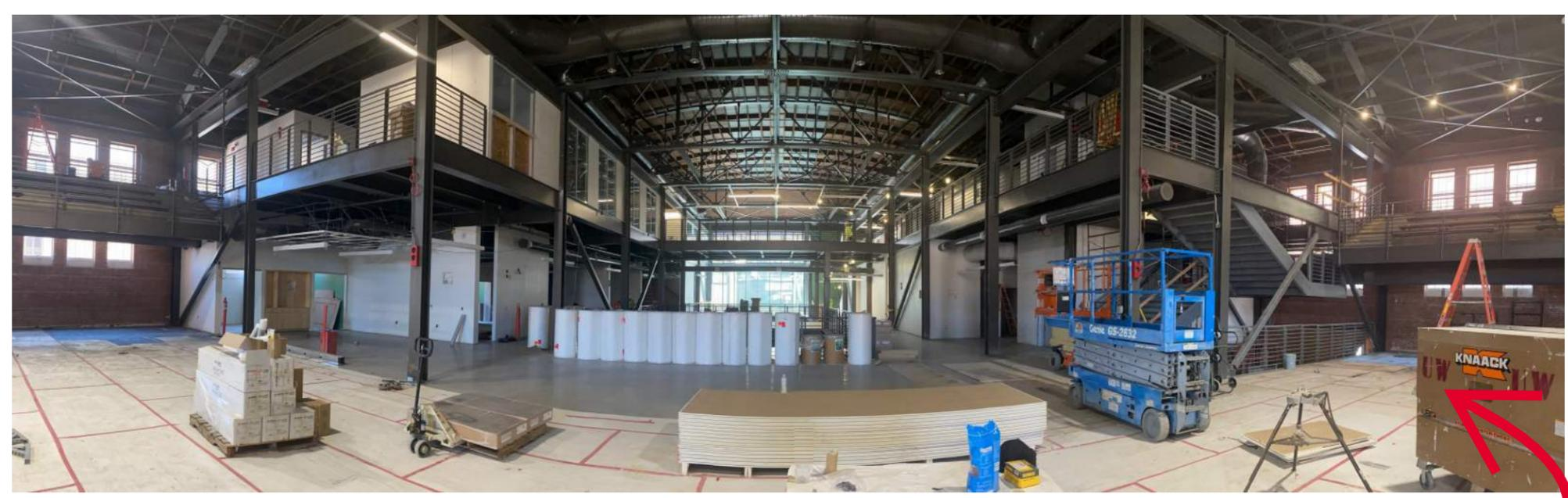
Inside the main entrance standing on the historic gym floor, looking south. Bleacher railings are installed on level 3, the staged materials are clearing off the historic gym floor this week, and aluminum windows are framing out on level 1.
