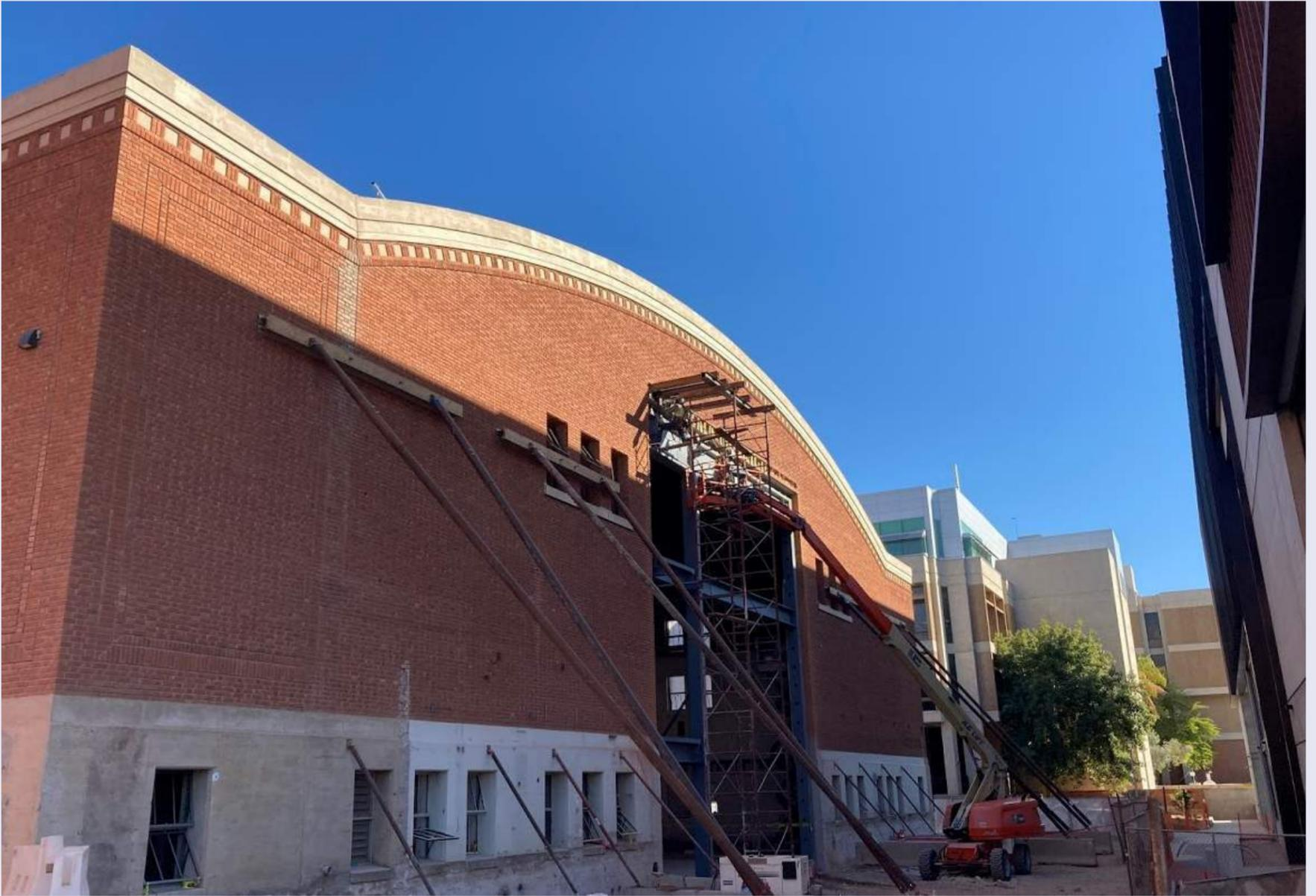
*Exterior view of the south side of Bear Down Gym with the new entrance which will connect to the new Bartlett Academic Success Center. Steel framing was installed to support the existing structure.*
